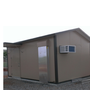
Electric Sub Station
