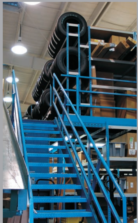
Shelving supported mezzanine with tire racks and long parts storage.
