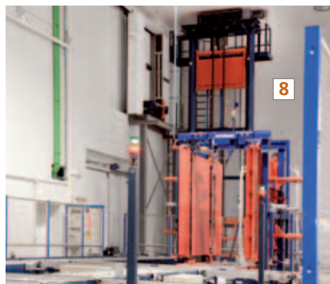
The roller or chain conveyors, automatic control station, compactor, elevators and security features all ensure an automatic, secure and high-capacity transport control.
