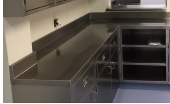
stainless steel countertops fabricated to drawings indicating backplash height, raised edge and field condition requirements
